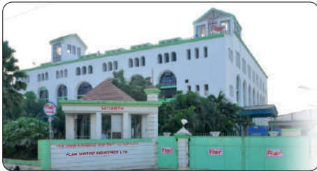
Daman - Plastic Facility
