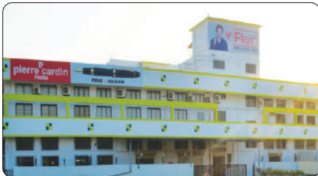
Daman - Plastic Facility
