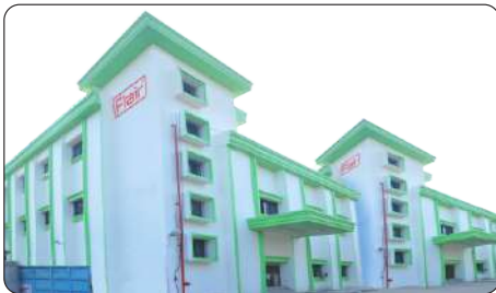
Daman - Plastic Facility
