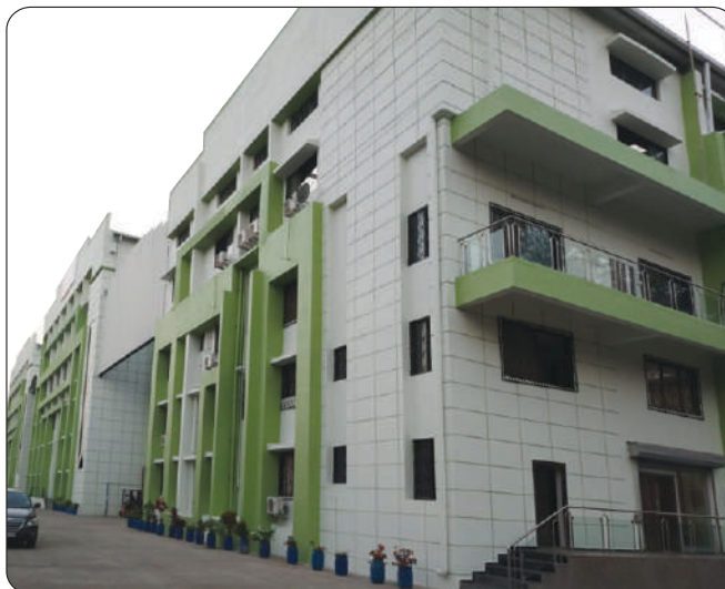
Daman - Plastic Facility
